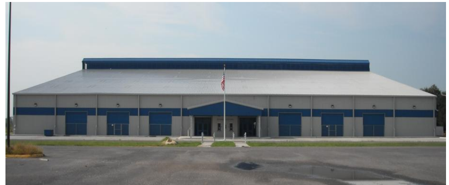
The dark blue areas you see are roll-up doors on the north side. (Directions are on the left side of this page.)
