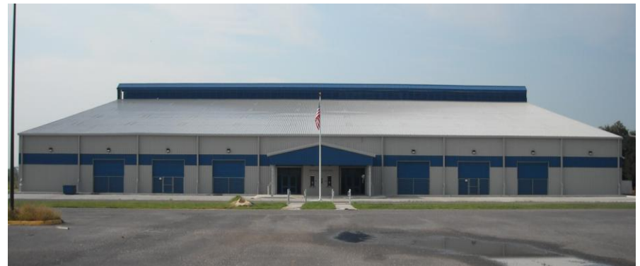
The dark blue areas you see are roll-up doors on the north side. (Directions are on the left side of this page.)
